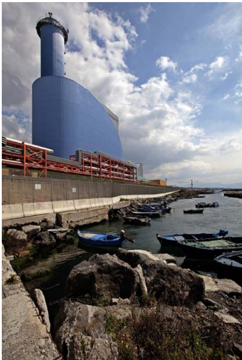
Naples Power Plant
