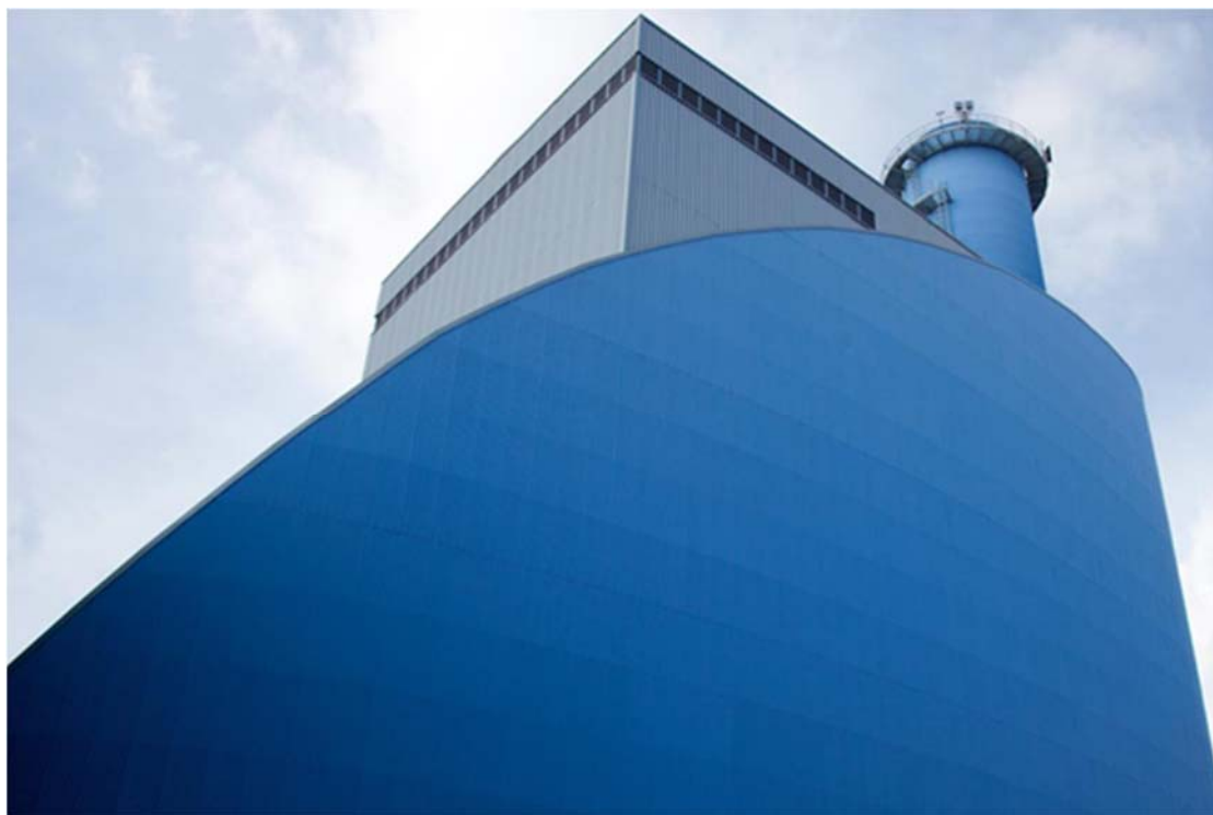
Napoli Power Plant
