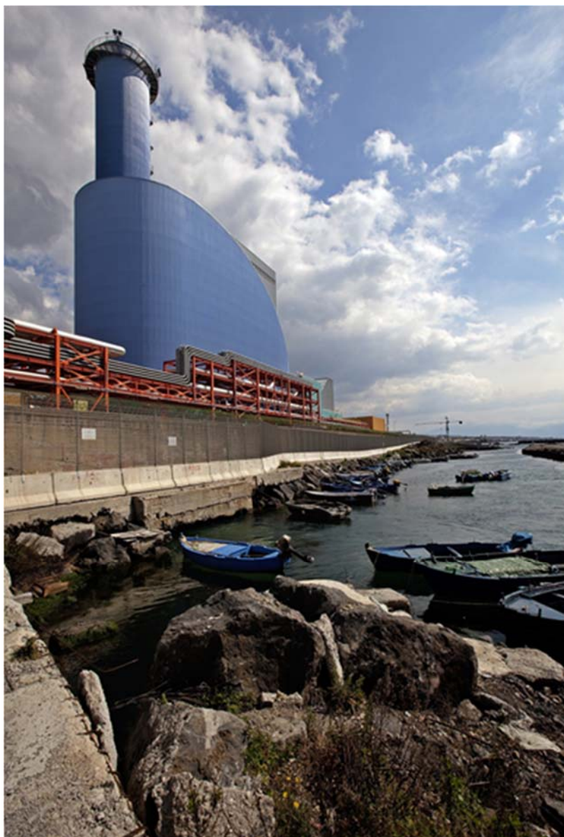
Napoli Power Plant
