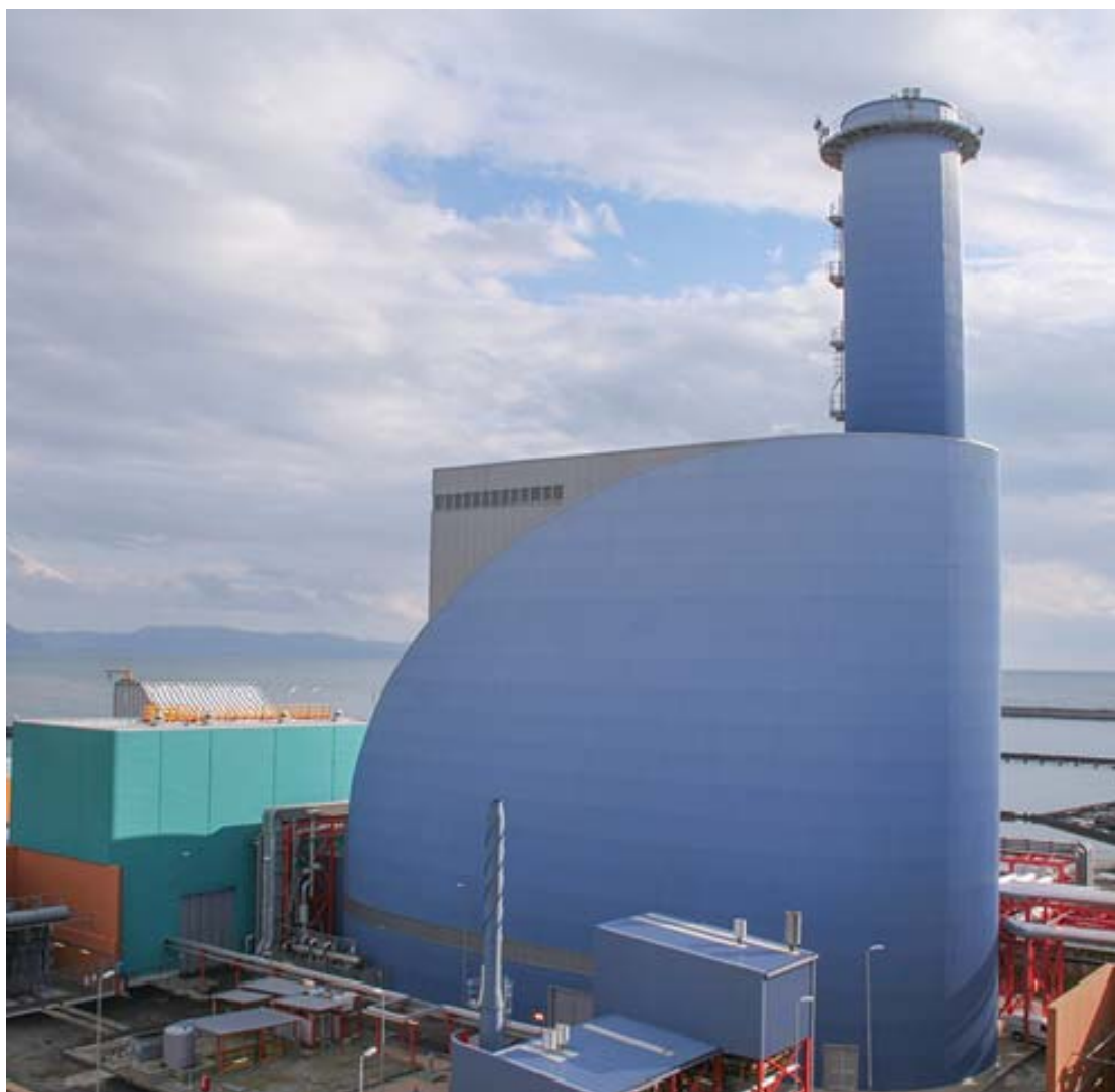
Naples Power Plant
