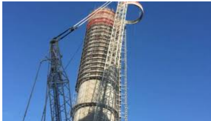
Vado Ligure plant – chimney stack demolition activities
