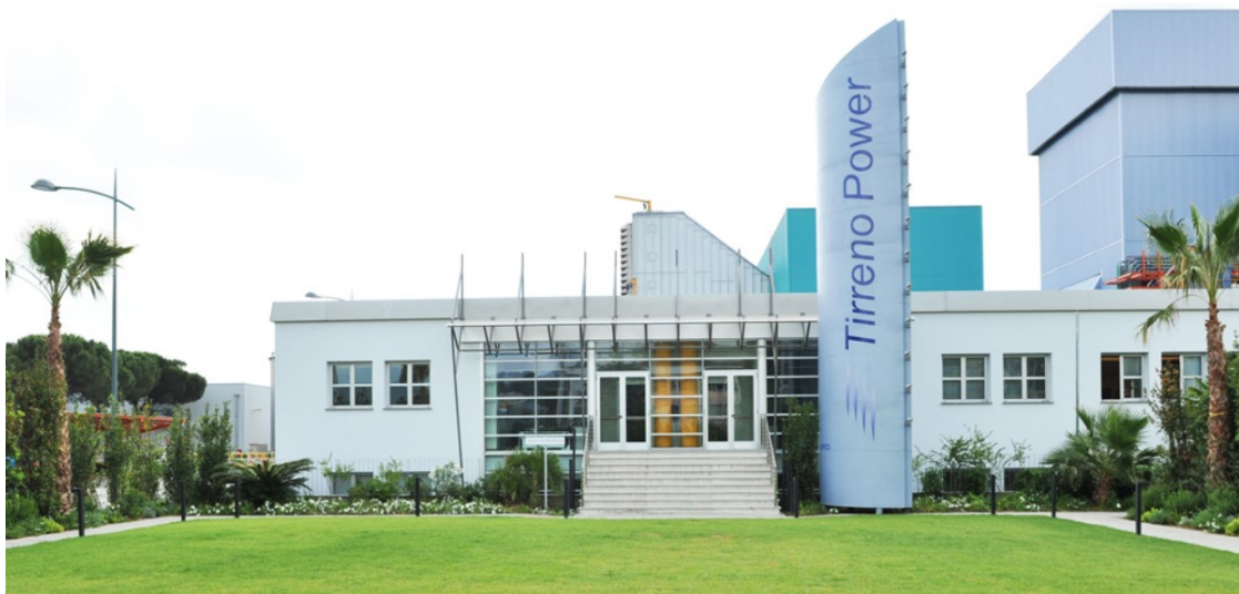
Vado Ligure Plant
